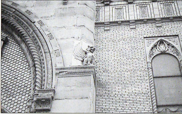
Detail of the former B'nai David synagogue on Elmhurst Avenue in Detroit, showing one of the winged creatures on its façade.
